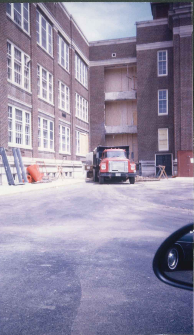
New Elevator Fall-1990
