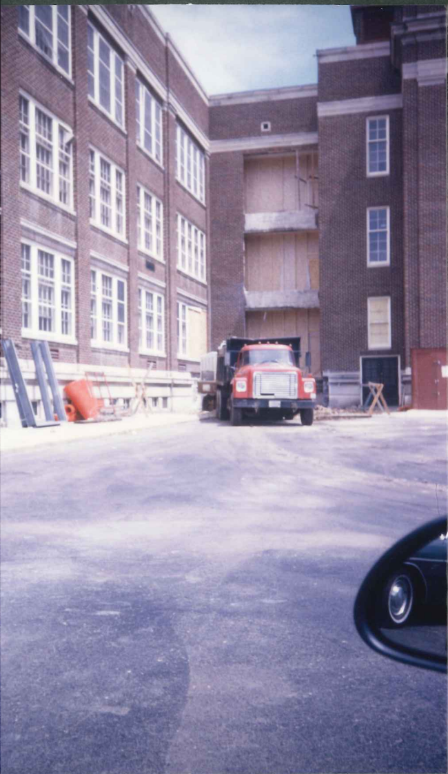
New Elevator Fall-1990
